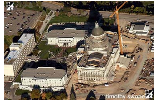
Renovation at the Utah State Capitol
